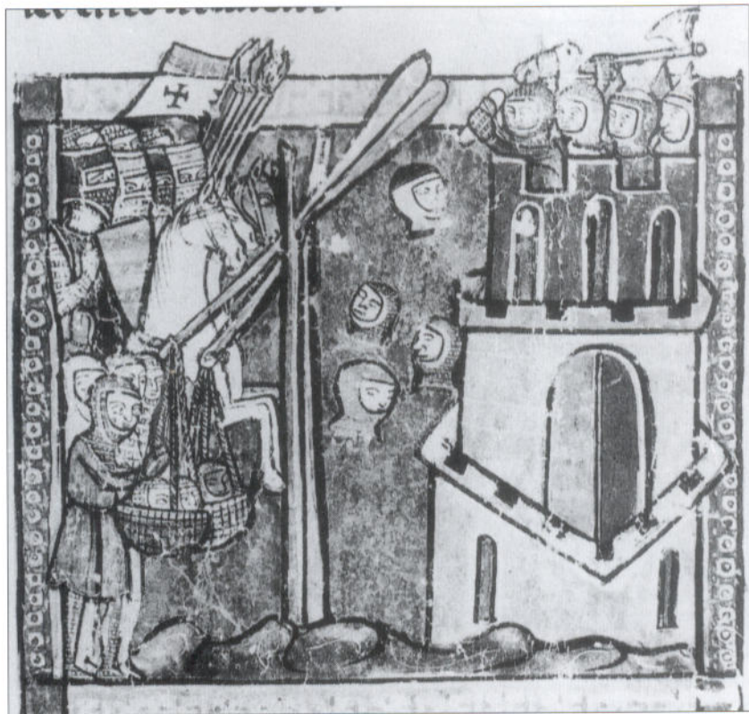
This early 13th-century French picture of Crusader siege machines hurling enemy heads into Nicea shows what might be a largely misunderstood early form of the counterweight trebuchet. There are clearly no teams of rope-pullers, while the bulging ends of the beam-slings might be an artist's attempt to indicate an early form of fixed counterweight. (Ms. Fr. 2630, f.22v, Bib. Nat., Paris)
