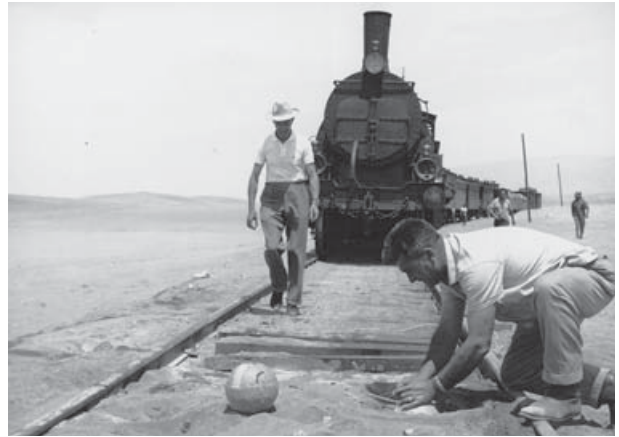
Above: Not a wartime demolition! The special-effects crew of David Lean's Lawrence of Arabia prepare to mine a train for one of the film's most dramatic scenes. (Author's Collection)
