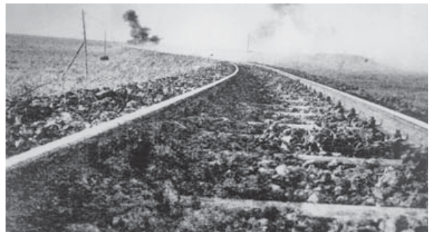
Below: A wartime photograph of a mine exploding on the Hejaz Railway. This appears to be a 'tulip mine', which were designed to bend the rails out of shape in order to make it more difficult for repair parties. Some of the raids on the line entailed the detonation of dozens of charges. (IWM Q60020)
