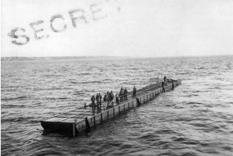
An assembled 2X30 pontoon causeway section. (Image provided by Andrew Hussey, Manston, UK)
