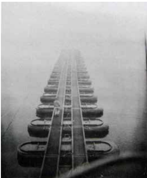
Assembled treadway bridge at Narragansett Bay, 18 March 1943. (source as previous image)
