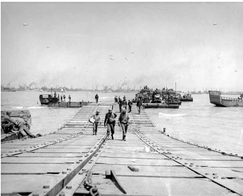
Civil Engineer Corps officers from the 111th Naval Construction Battalion walking across a double-wide causeway at Omaha Beach. (National Archives and Records Administration)
