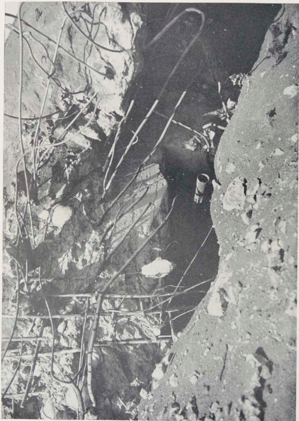
Reinforced Concrete Fill Box
